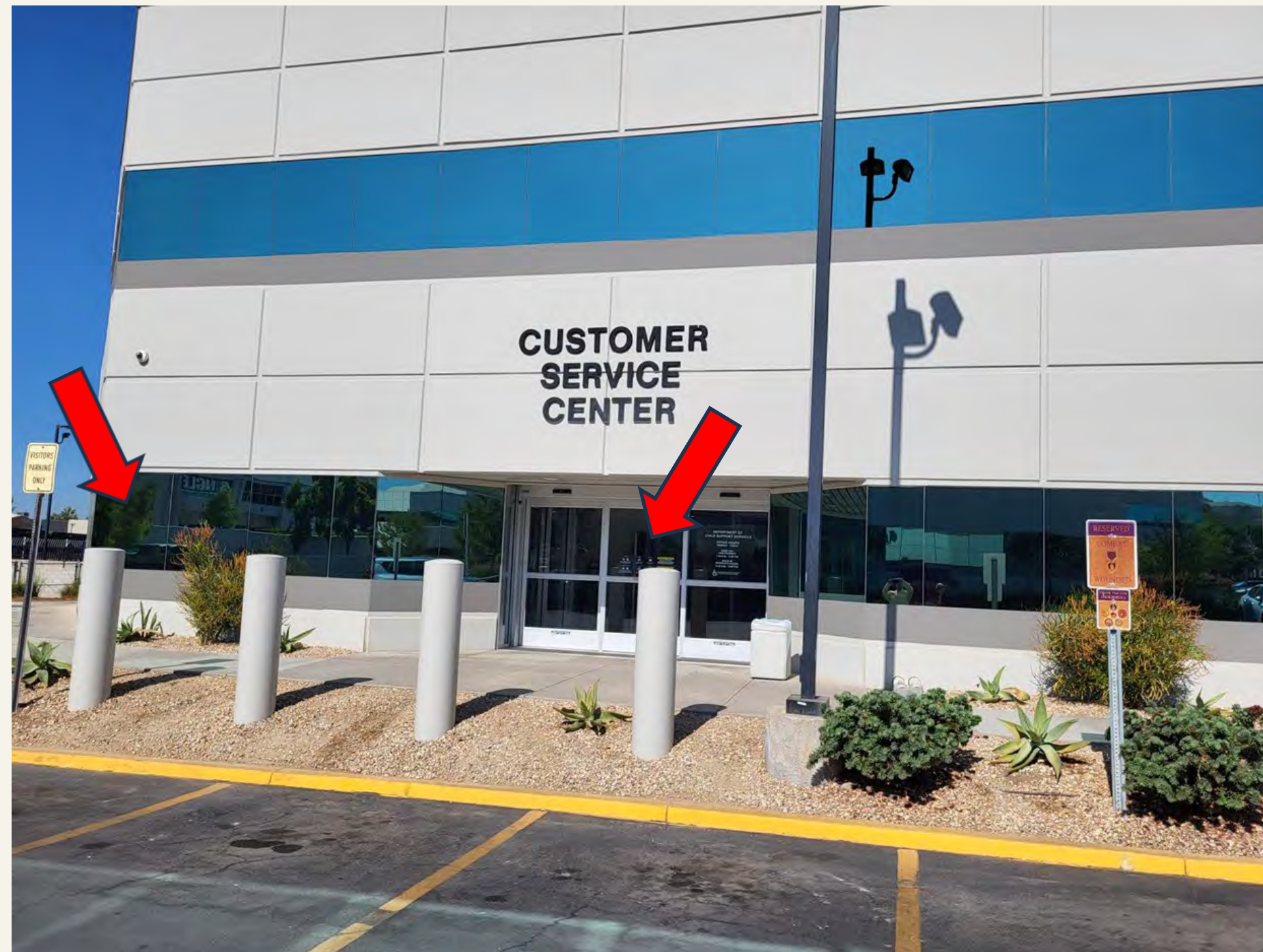
Bollards were placed in front of the Customer Service Building
